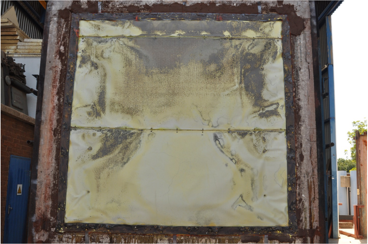
Figure 3.12: Exposed side of specimen wall after removal from the SANS 10177 – 2 facility
