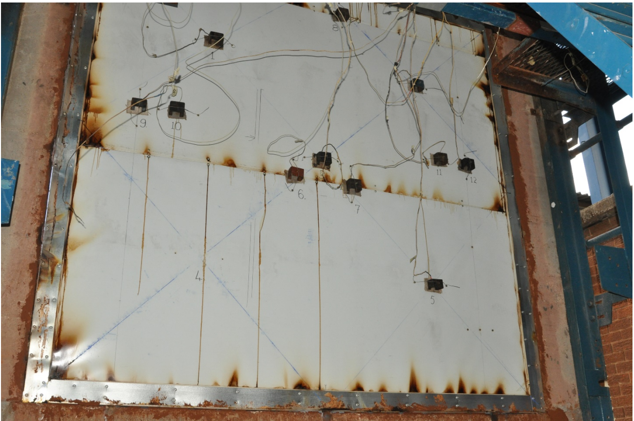
Figure 3.13: Unexposed side of specimen wall after removal from the SANS 10177 – 2 facility
